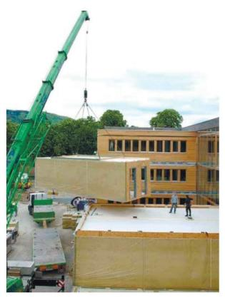
Figure 3 Examples of constructions; apartment building, modular system.
