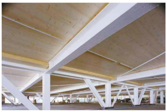
Figure 3 Examples of constructions; multi-storey car park.
