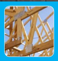
Prefabricated structural members assembled with punched metal plate fasteners (EN 14250);
